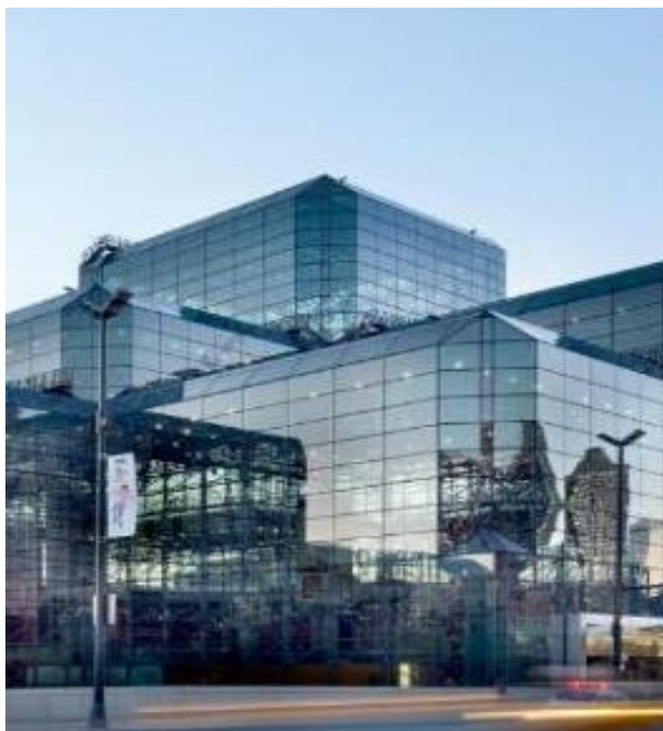
Figure 4. The Jacob K. Javits Center, Newly Completed Full Replacement of Exterior Glazing with Bird Friendly Material (TF < 25) (Source: FXCollaborative)
