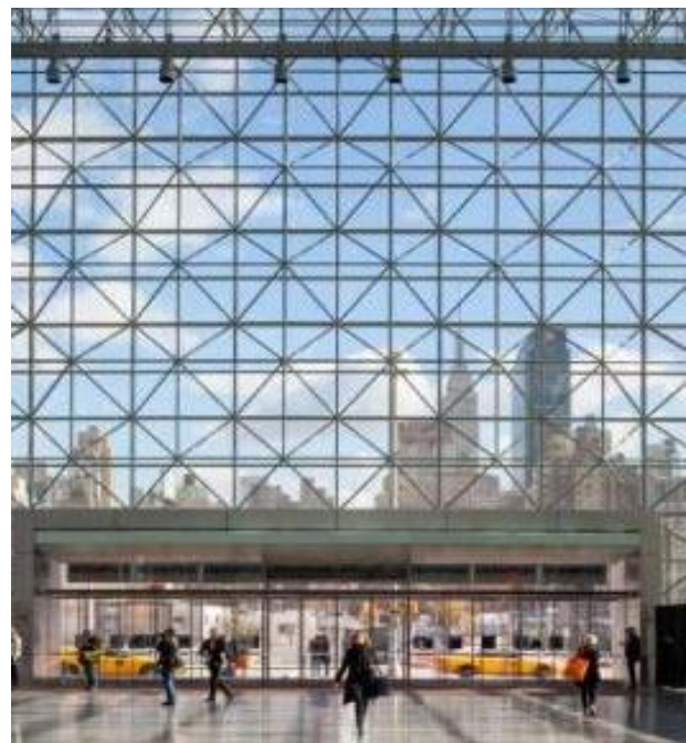
Figure 4. The Jacob K. Javits Center, Newly Completed Full Replacement of Exterior Glazing with Bird Friendly Material (TF < 25) (Source: FXCollaborative)
